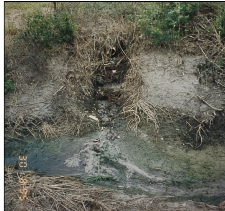
Drainage ditch in the Tres Palacios watershed is used as a sewer.
