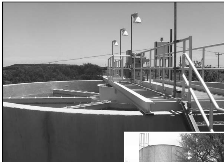
Lometa Water Treatment Plant
