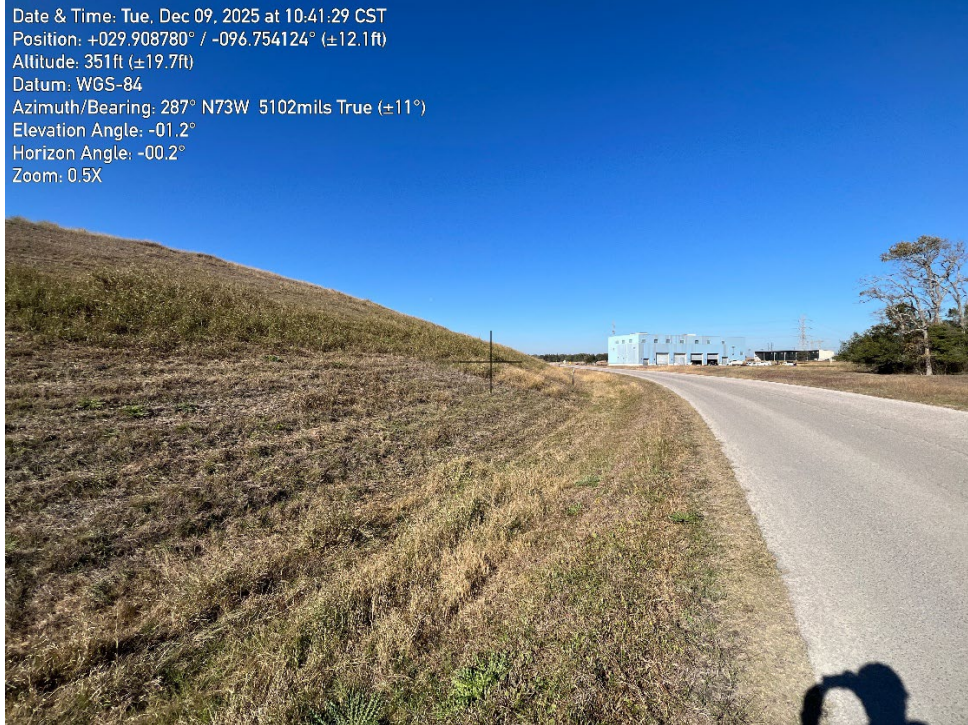
Photo 1 – Cell 1 North Embankment, Facing Northwest
