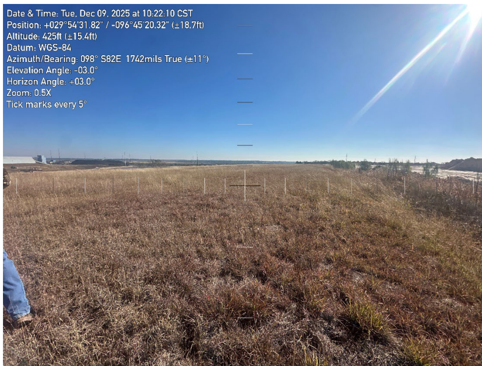
Photo 2 – Cell 1 Capped Area (left) and Landfill Material (right edge), Facing Southeast
