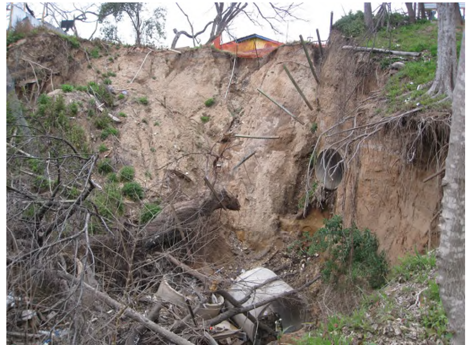
$1.9M Tillery St. Outfall Repair
