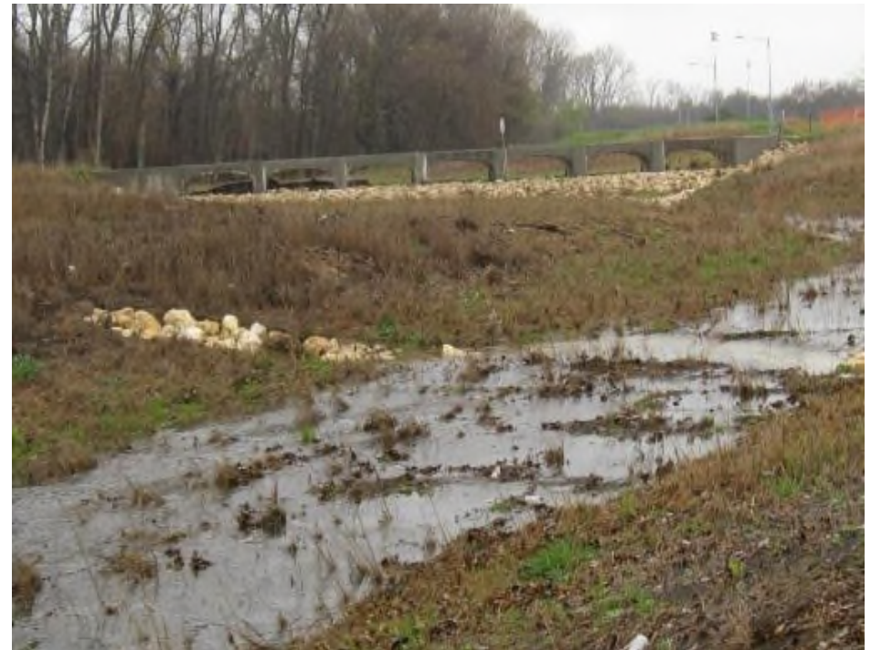
Roy Guerrero Park: Original pedestrian bridge
