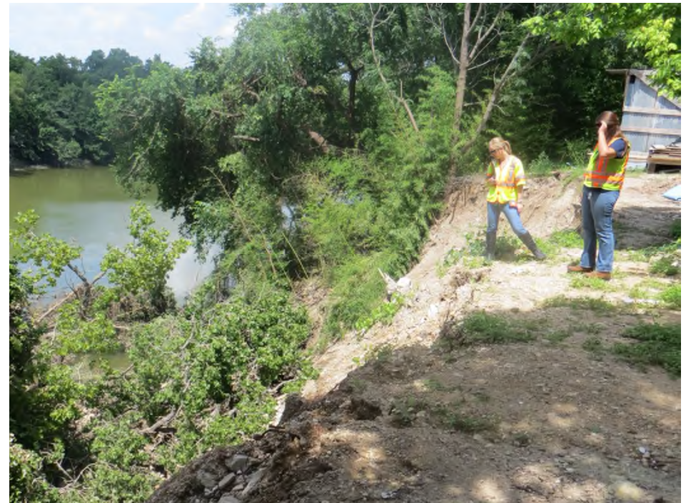
Home threatened after bank failure, May 2015
