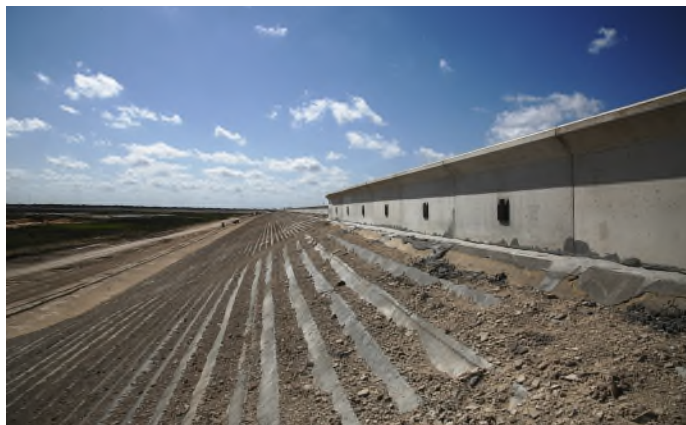
Custom-built concrete parapets along the top of the embankment will prevent wave action that could damage the reservoir.
