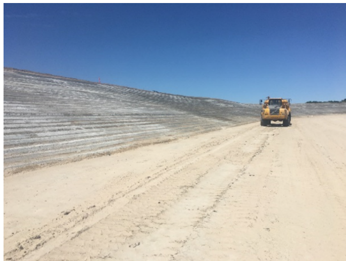
A truck waters down the sides of the new reservoir, which is strengthened with soil cement, during construction in 2017.
