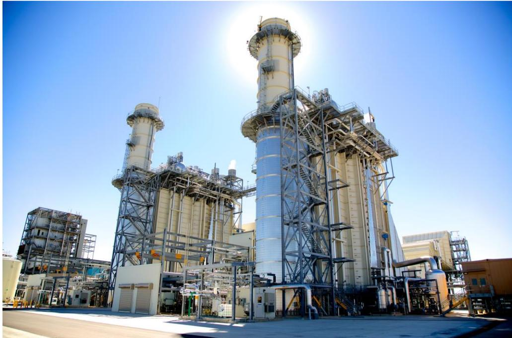
The Thomas C. Ferguson Power Plant is a natural gas-fired, combined-cycle plant in Horseshoe Bay, Texas, near Lake LBJ. The highly efficient plant can generate between 510 and 580 megawatts of power, helping LCRA and its wholesale electric customers provide electricity to about a million Texans.
