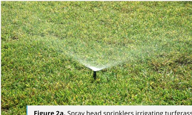
Figure 2a. Spray head sprinklers irrigating turfgrass.
