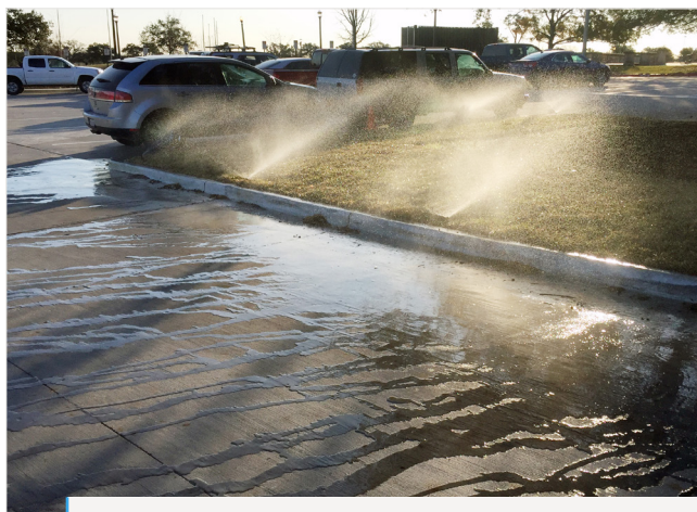
Figure 1. Example of runoff from spray head sprinklers.
