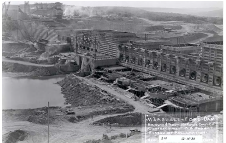
Mansfield Dam construction, 1938. (LCRA Archives W00170)
