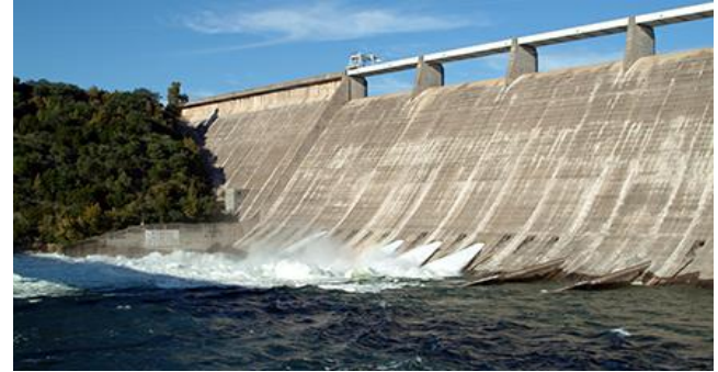
Mansfield Dam during flood operations in May 2016.
