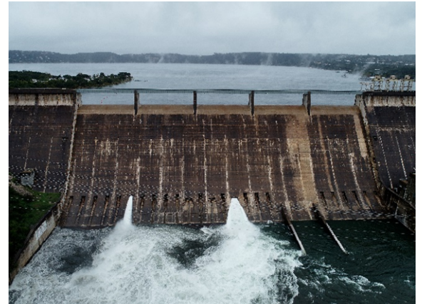
Mansfield Dam during flood operations in October 2018.
