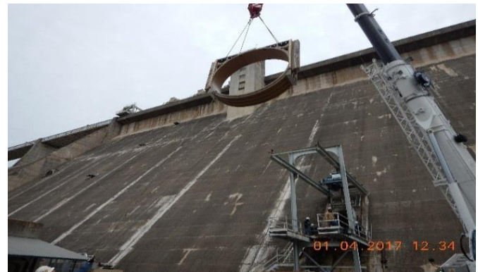
Mansfield Dam rehabilitation project, January 2017.
