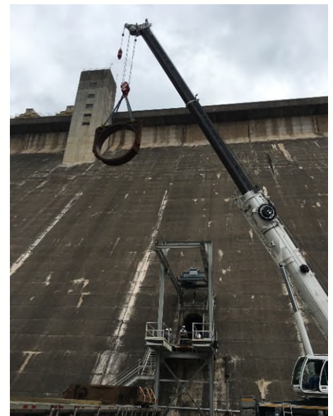
Mansfield Dam rehabilitation project, April 2019.
