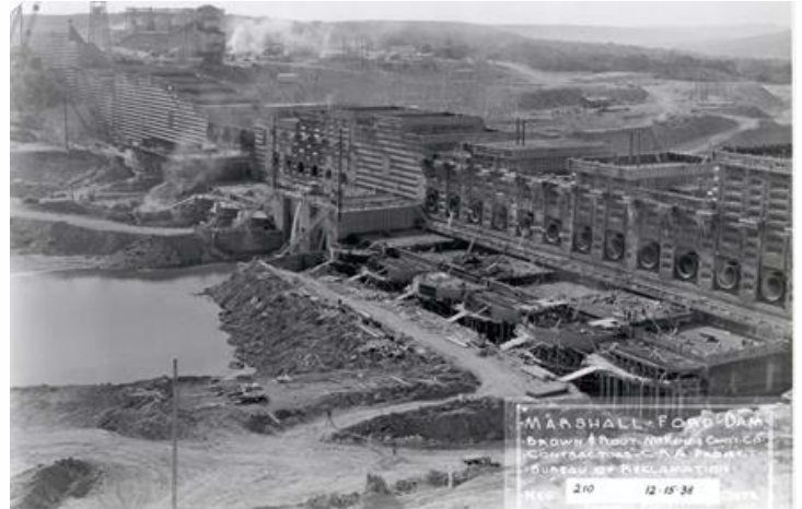
Mansfield Dam construction, 1938. (LCRA Archives W00170)
