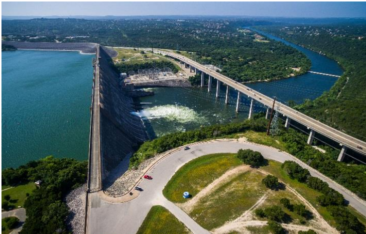
Mansfield Dam during flood operations in May 2016.
