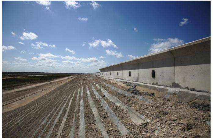
Custom-built concrete parapets along the top of the embankment will prevent wave action that could damage the reservoir.
